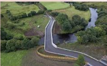
The new Mullantiboyle Bridge in Glenties
