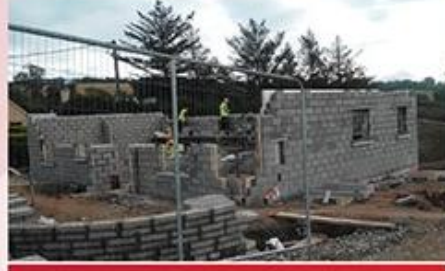
Houses under construction in Manorcunningham
